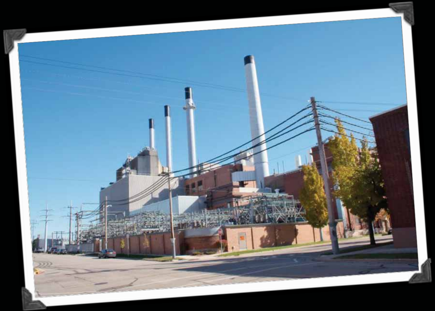
Madison Gas and Electric Blount Street Station
